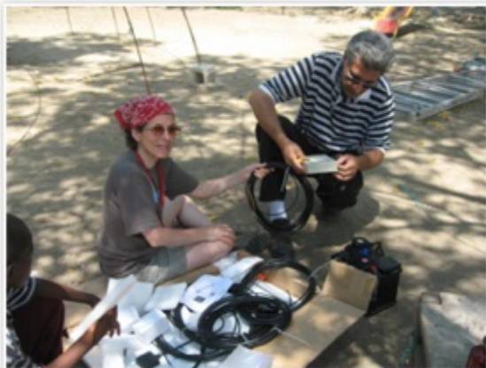
Solar panel being assembled
